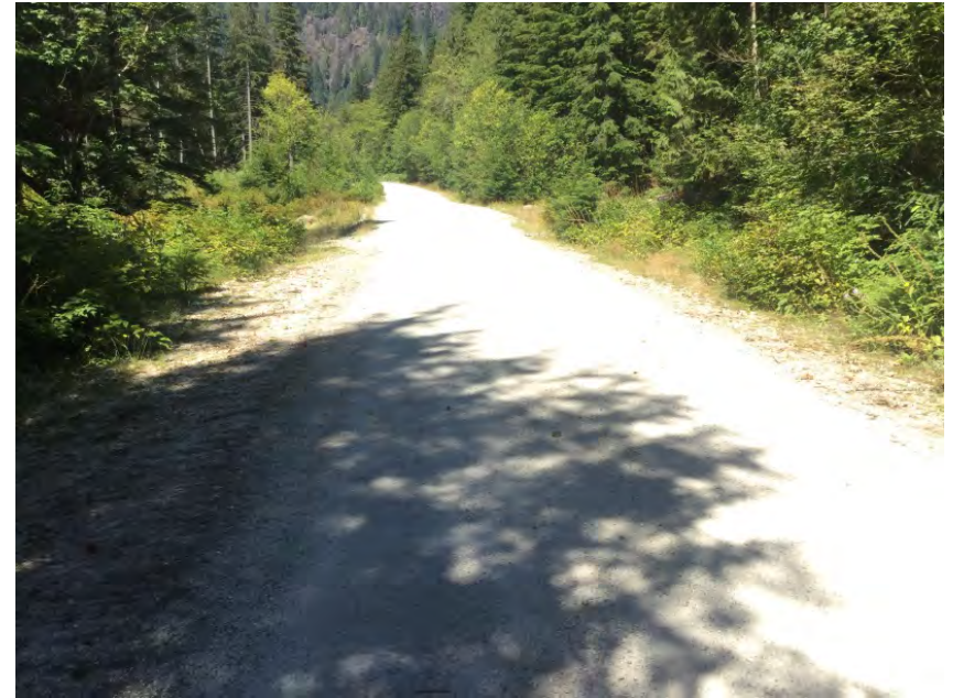
Roadway Over Culvert
