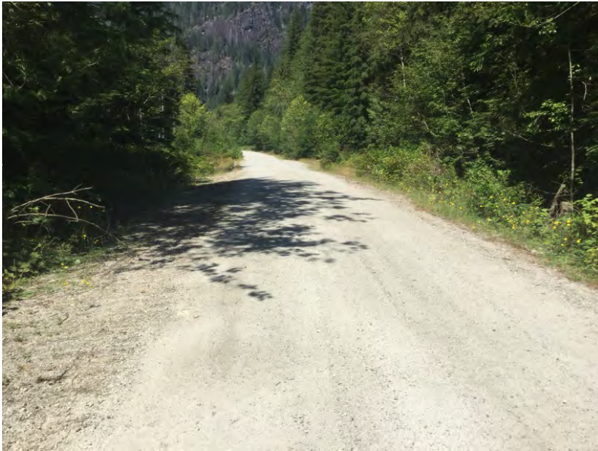
Left Approach Facing Culvert
