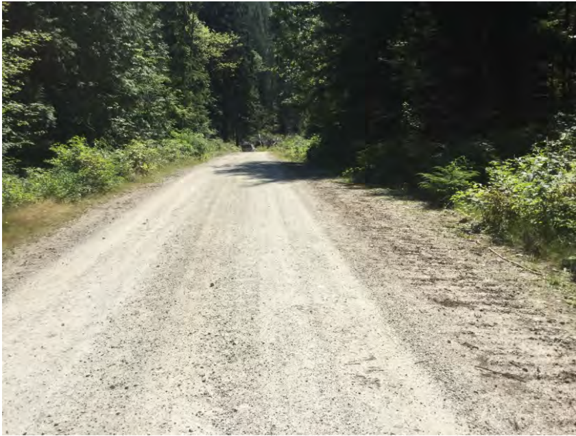
Right Approach Facing Culvert
