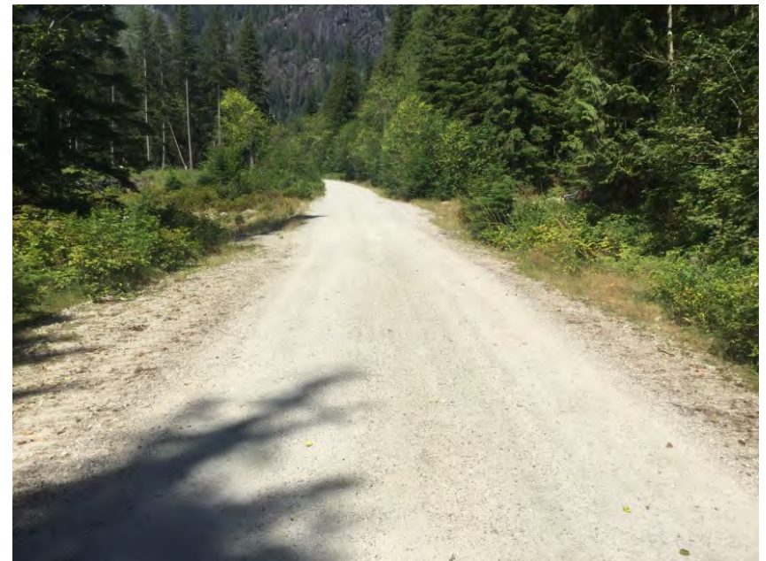
Right Approach Facing Away From Culvert
